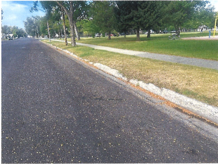
Deteriorated curb and gutter at Highland Park.
