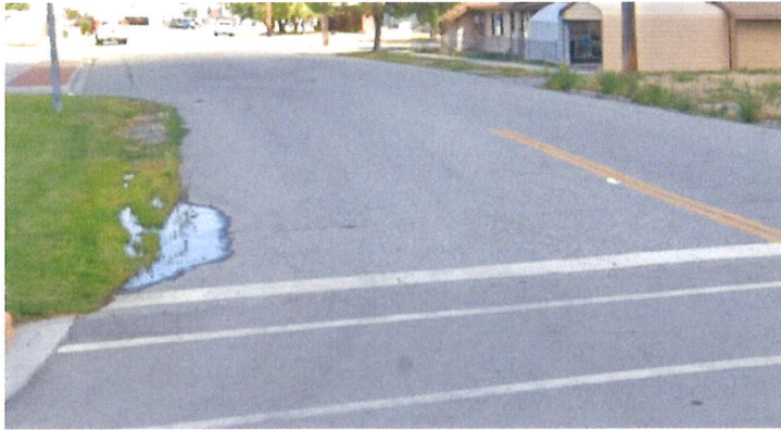
Improper drainage and missing curb, gutter or sidewalk on Fifth Avenue South near 27 th Street, right at the entrance to Downtown Billings.
