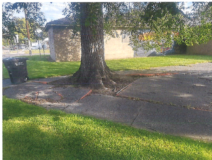
Damaged, unsafe sidewalks in South Park.
