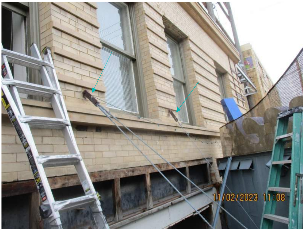
Figure 18: Cable Tie Back Connections at Exterior Wall
