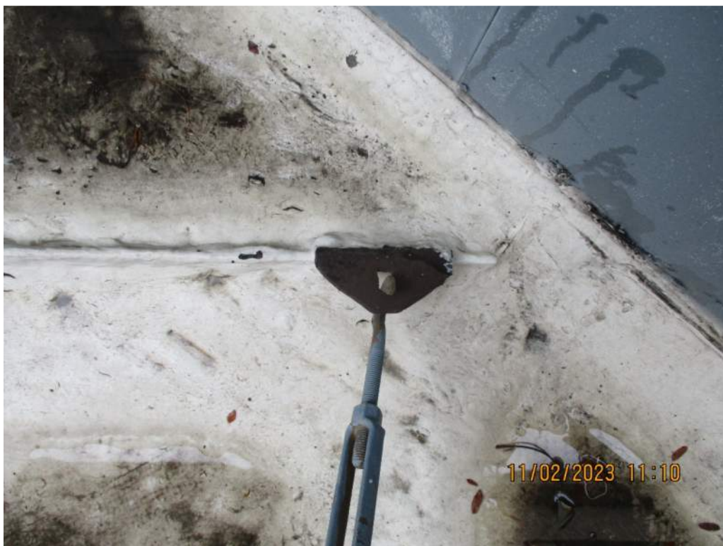
Figure 17: Cable Tie Back Connection at Roof Level
