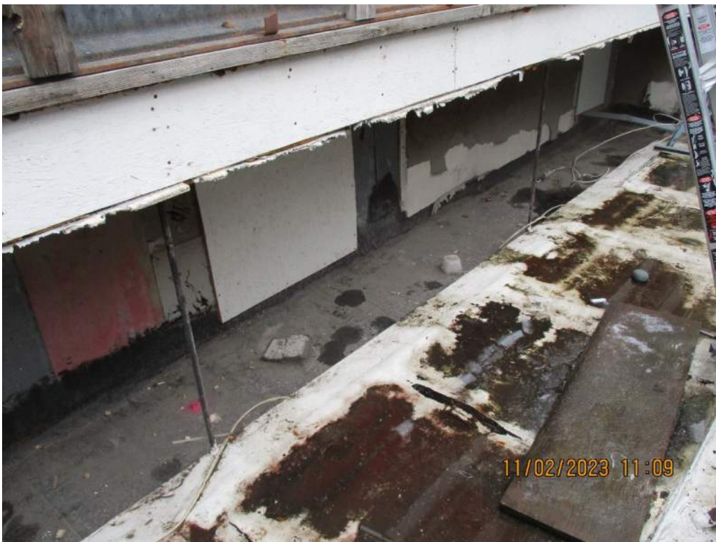
Figure 11: Deteriorated Built-Up Roofing at South End of Marquee Along Transition to Internal Gutter
