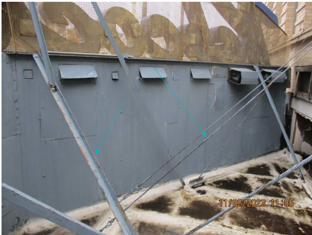
Figure 16: Marquee Support Cabling and Angle Iron Bracing
