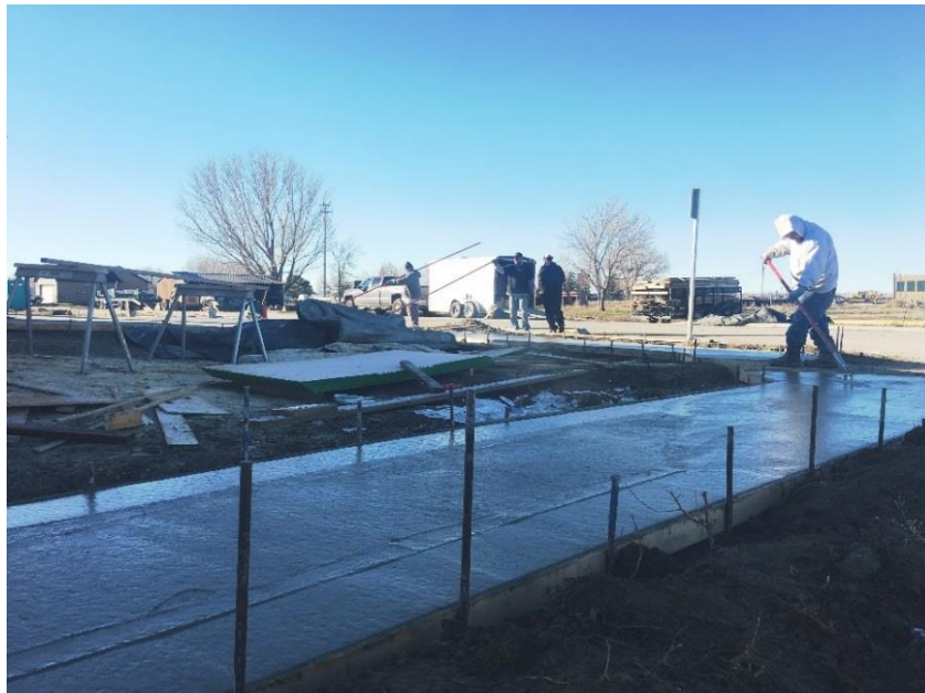
Image 1.1 Construction crews building boulevard sidewalks as a requirement for a new subdivision hence preventing increased installation costs in the future
