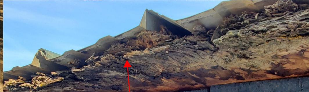
Do NOT include rotted deck in Base Bid. Upon demo of old metal roofing, call Owner's Rep for documentation, pricing & approval of decking replacement. Added Costs will be handled as a Change Order.
