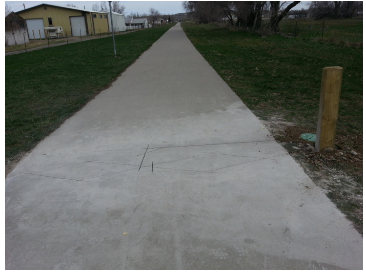
The Kiwanis Trail permanent counter after installation
