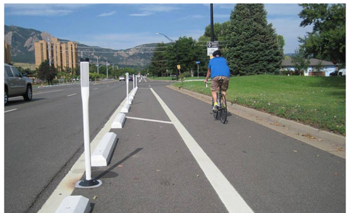
This Boulder, CO, one-way separated bike lane uses flexible posts and curbed intersection treatments to separate bicyclists from motor vehicles.
