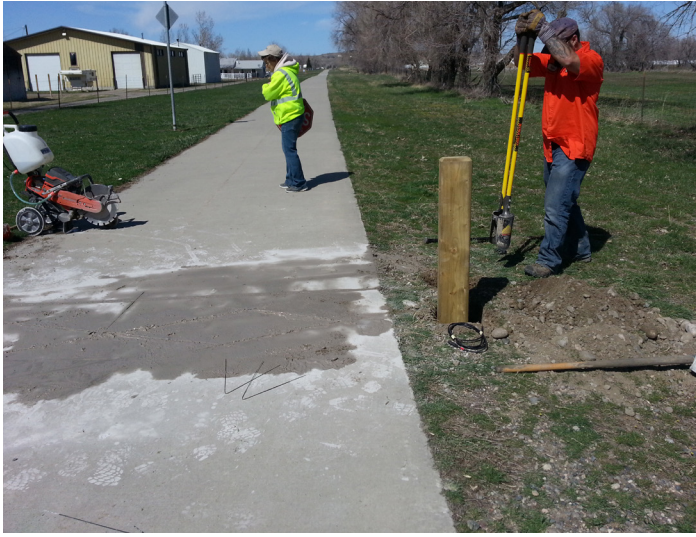
Permanent inductive loop and infrared counter being installed at Kiwanis Trail
