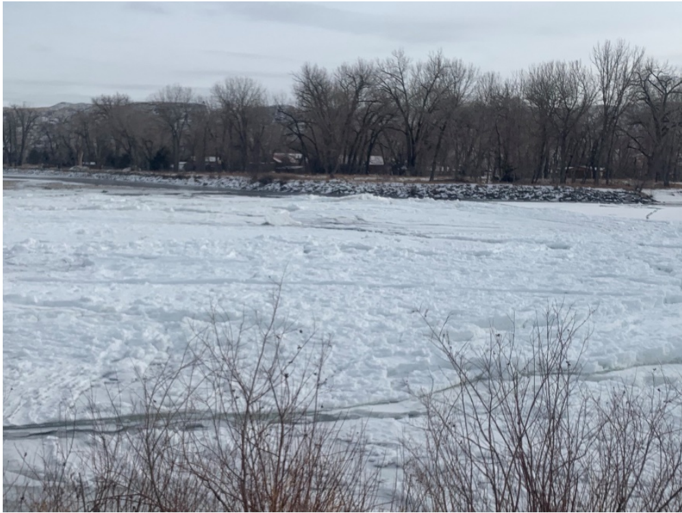
Picture of river today at site of new intake
