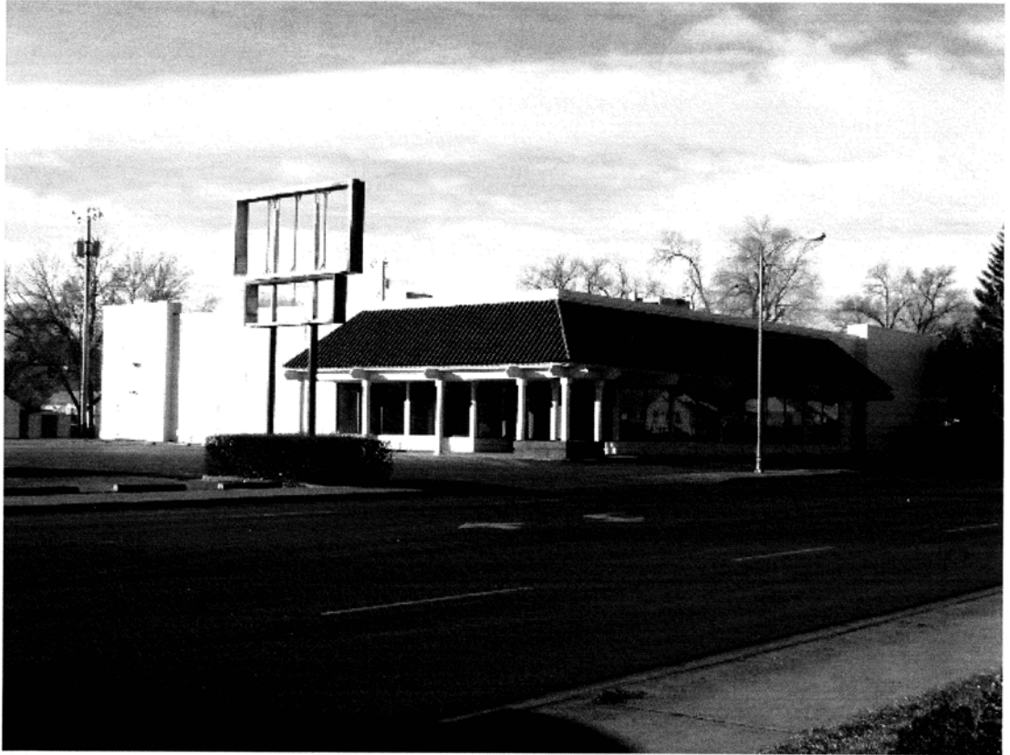
EXISTING BUILDING – 708 BROADWATER AVENUE PROPOSED FUTURE HOME OF: ARTHRITIS AND OSTEOPOROSIS CENTER
