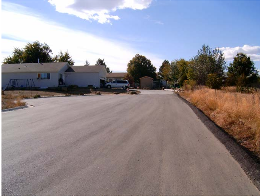
Looking west from along the frontage of the subject property on Saturn Drive.
