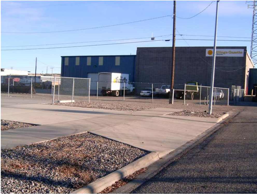
Looking south from 22 nd Street at existing structure.
