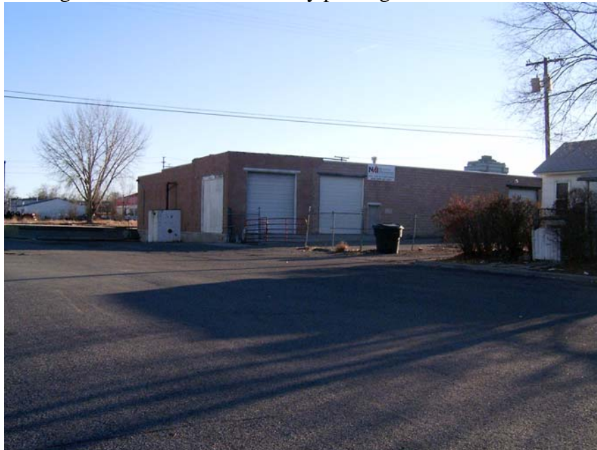
Looking south from 22 nd Street and 6 th Avenue North.
